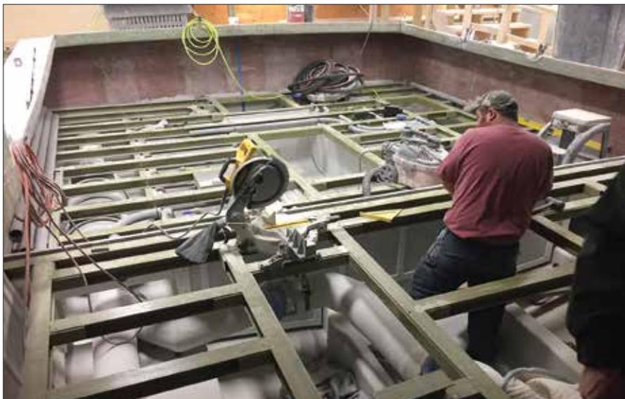
**Left**—The support grid of beams and stringers prior to deck installation reveals the mechanical systems and ample tankage space below the broad, open cockpit. **Right**—Full-size mock-ups helped inform final decisions like the one to not carry two Rocna anchors on bow rollers.
